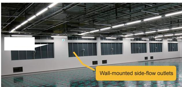
Figure 11: Side-flow Air Conditioner Outlets
