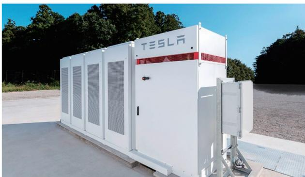
Figure 16: Powerpack installed at Shiroi DCC
