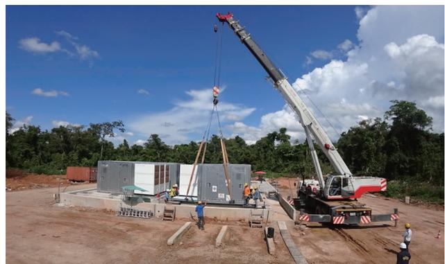
**Figure 3: Installation of a Module by Crane**
